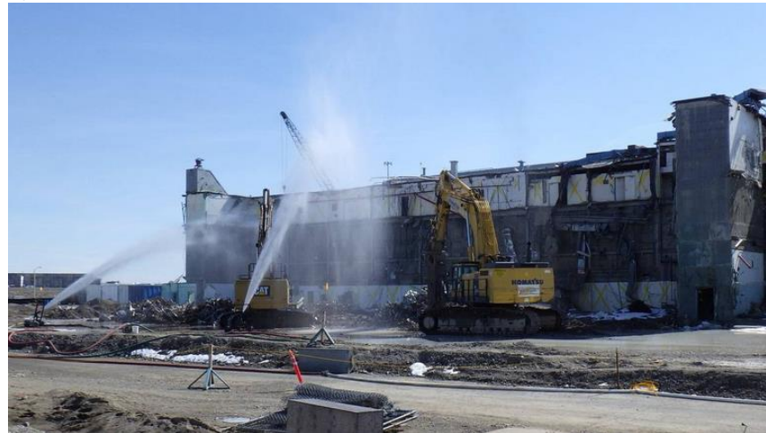
Cleanup mission at Hanford that was stalled
