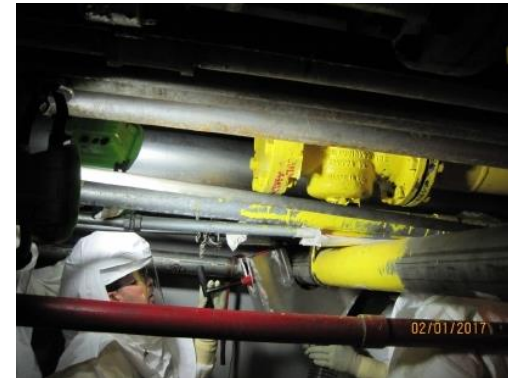
Contaminated Pipes at Hanford
